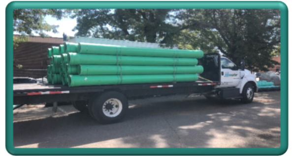
Pipe delivery to the project staging area
