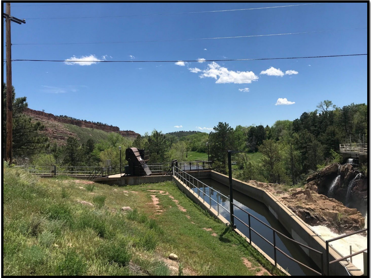
Figure 7. Loveland Water and Power Big Thompson River intake structure.
