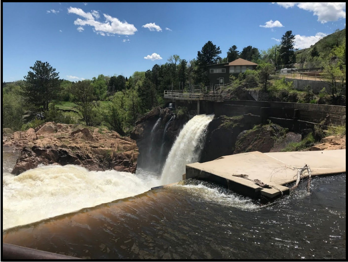
Figure 11. Big Thompson River control structure (foreground) and Home Supply Canal control structure (background).
