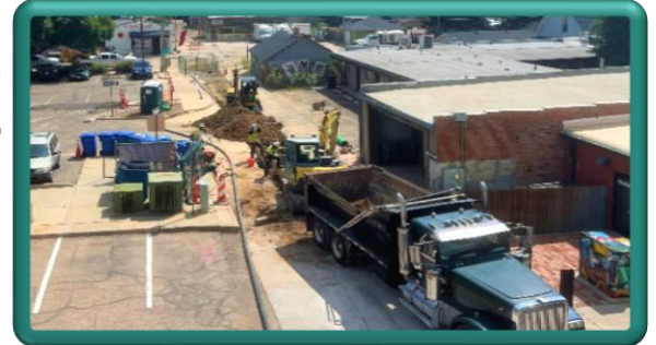
Construction progress west down Sweetheart Alley; Washington Avenue at top
