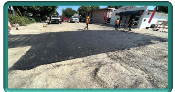
Asphalt pavement repair across Washington Avenue prior to reopening
