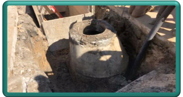
Removal of existing wastewater manhole in Sweetheart Alley
