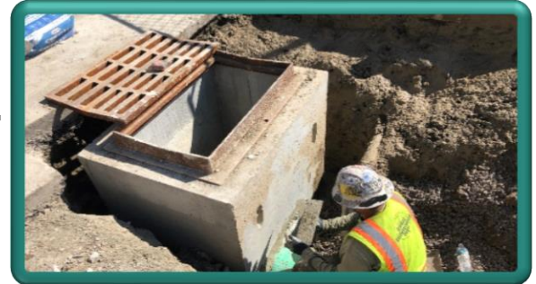
New storm drain inlet at Washington Avenue
