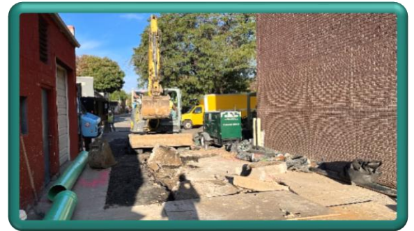
Pavement removal in narrow section of alley at Jefferson Avenue
