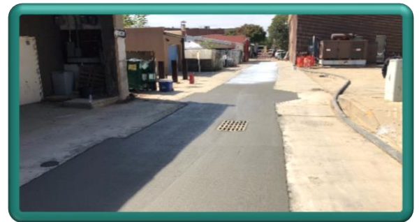
Pavement replacement in alley, west of Washington Ave
