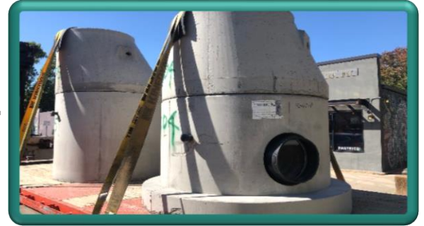
Concrete manhole sections to be used for both storm drain and wastewater pipe junctions
