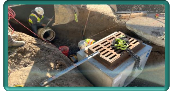
New storm inlet installation in Jefferson Avenue
