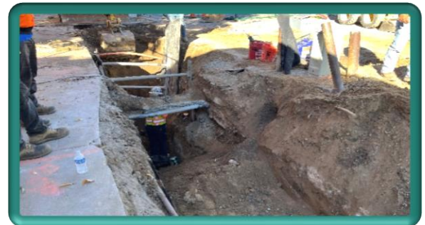
Open trenching through the alley, looking west
