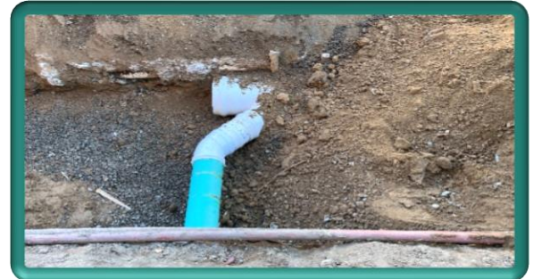
Reestablishment of existing roof drain lateral to the new storm drain
