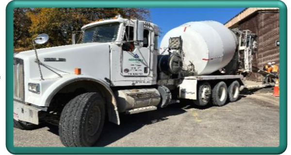
Concrete pavement placement in alley adjacent to Jefferson Avenue
