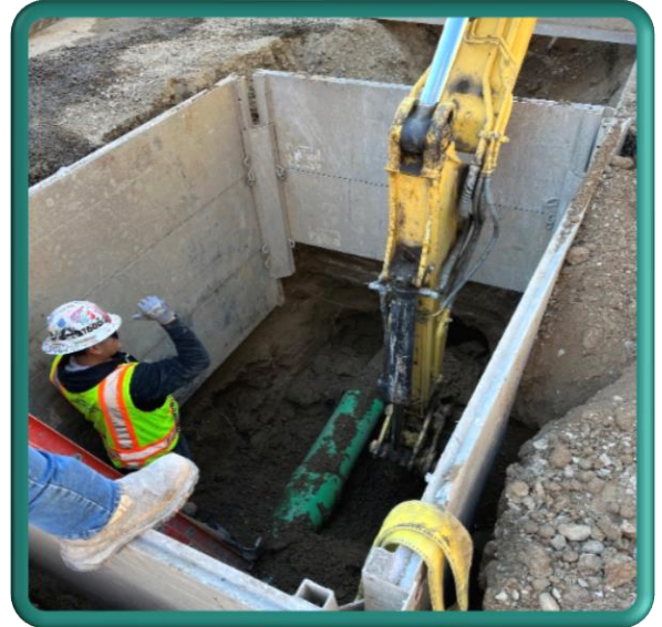
Excavation of trench looking west in Jefferson Avenue
