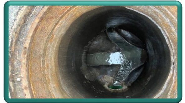
Inspection of new connection to existing manhole
