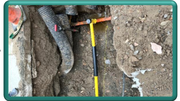
Re-routing of existing gas line to facilitate new sewer installation
