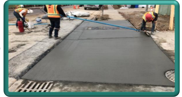
Pavement repair in Washington Avenue
