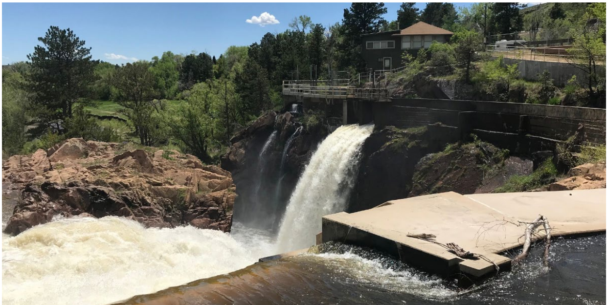
Loveland Water & Power drinking water intake. The Home Supply Canal visible on the far side of the Big Thompson River.
